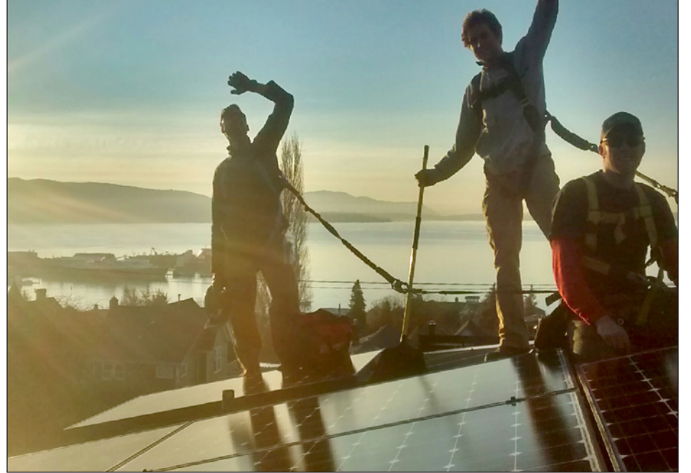
Western Solar Installers
